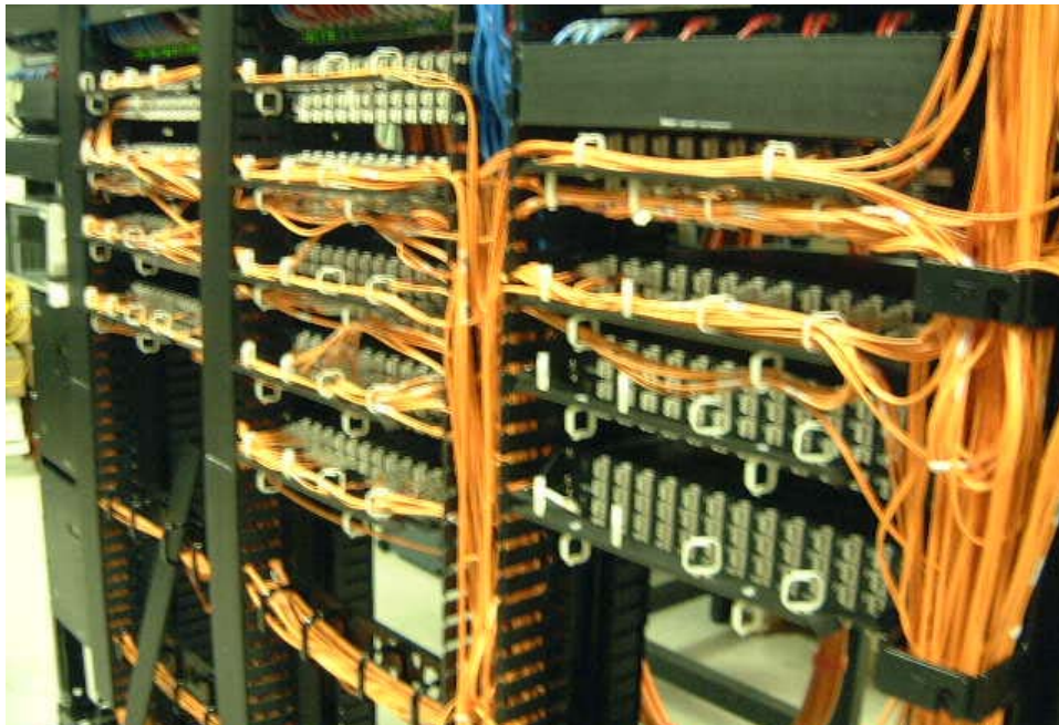
Figure 3-4 Patch Panel With Cable Guides
